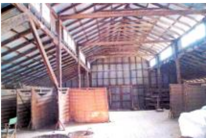
Wallandool Station shearing shed wool handling area.
